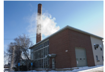
Central Heating Plant at USM Portland Campus
