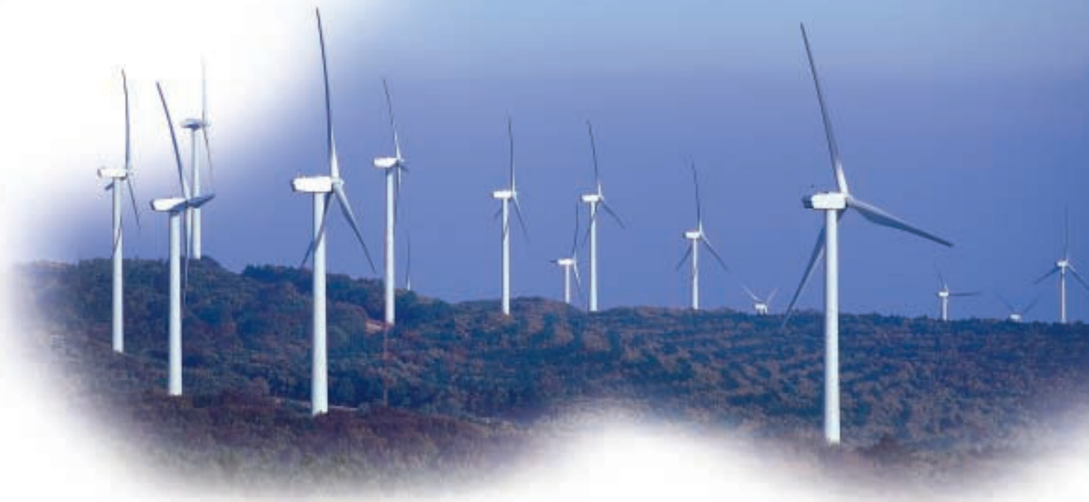
Escurillo, Spain 33 x 1.5sl, total capacity: 49.5 MW
